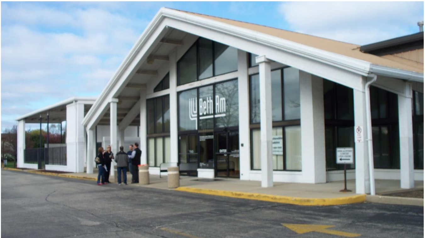
FIGURE 2: BUILDING FAÇADE WHEN IT WAS STILL OPERATING AS TEMPLE BETH AM
